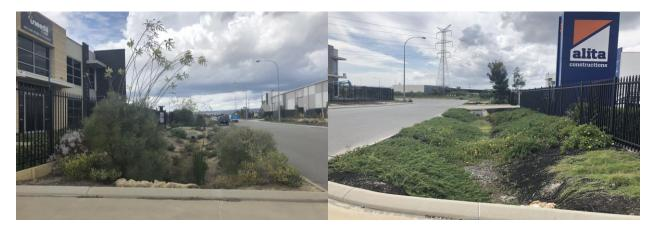
VEGETATED STORMWATER SWALE CONCEPT
